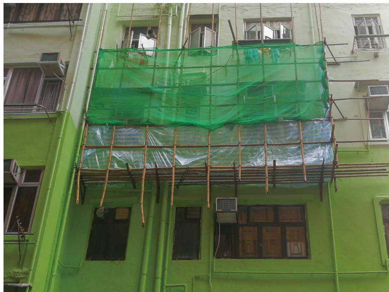
Figure 11: Truss-out bamboo scaffold
