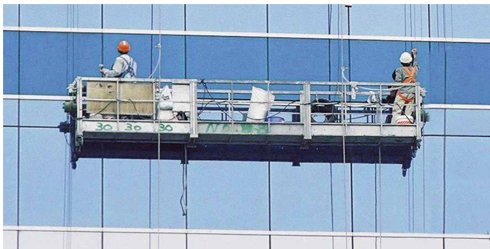
Figure 13: Suspended working platform
