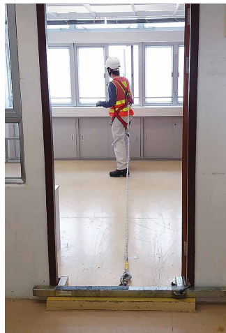
Figure 16: Transportable temporary anchor device
