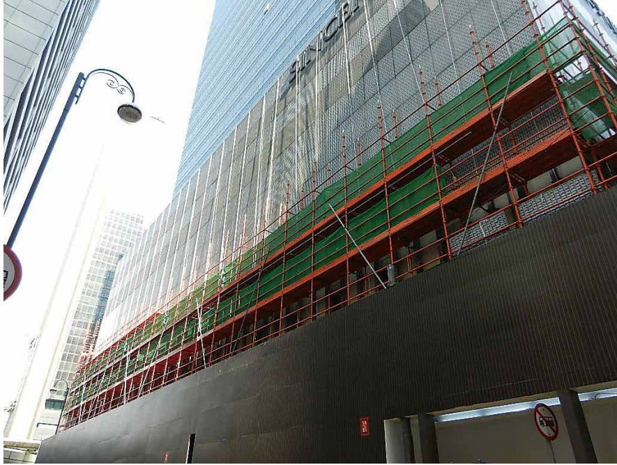
Figure 9: Independent tied metal scaffold
