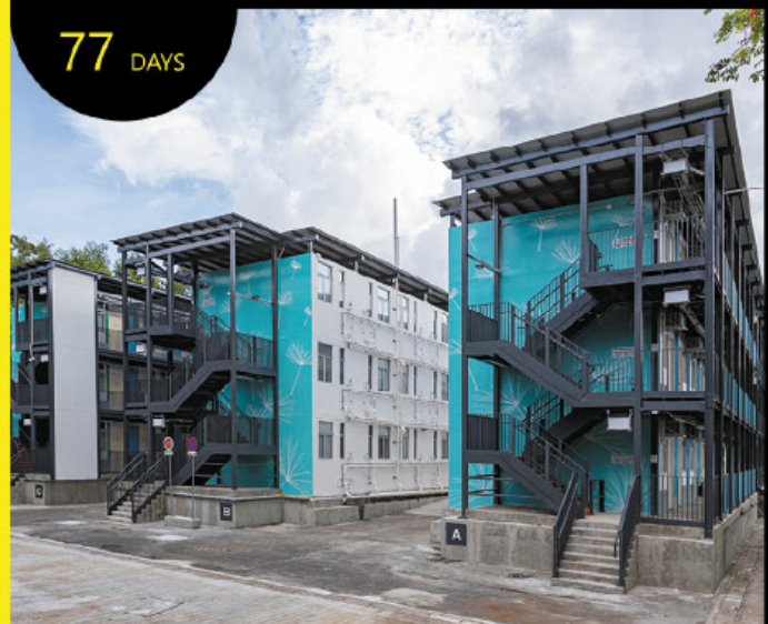
SAI KUNG OUTDOOR RECREATION CENTRE
